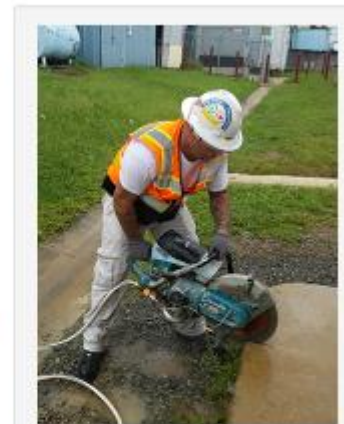
Applying water to a saw blade when cutting materials that contain crystalline silica — such as stone, rock, concrete, brick, and block — substantially reduces the amount of dust created during these operations.
